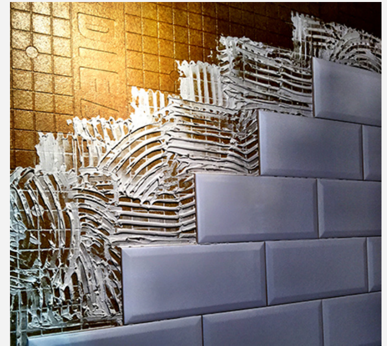
New Shower Construction Waterproofing and Air & Vapor Protection
