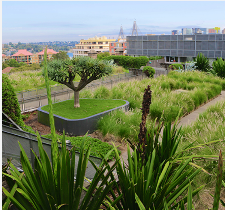
New Green Roof Construction
