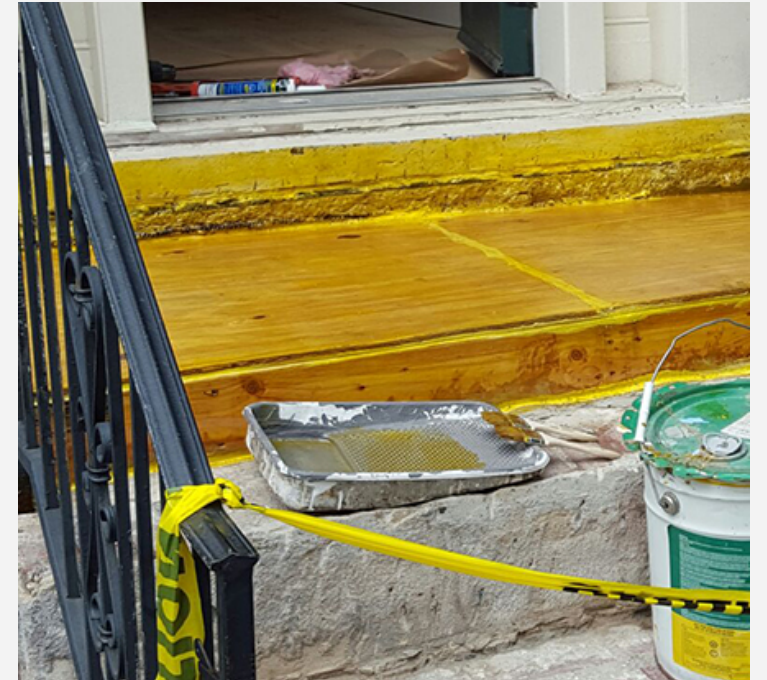
New or Existing Deck Construction and Repair
